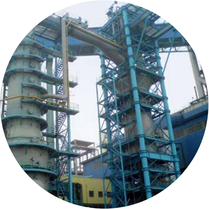
Xianghan blast furnace conditioning tower and scrubber
